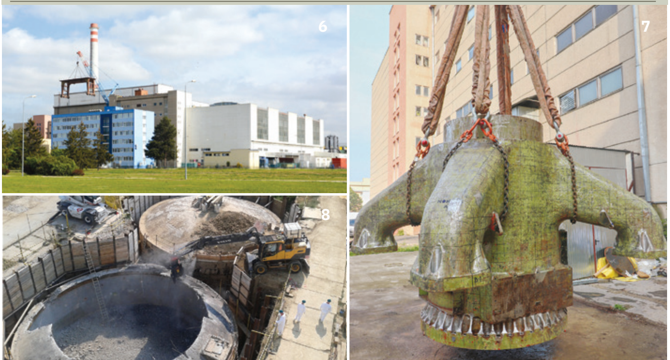
1. Dismantling of the electric generator in the turbine hall; 2. Fragmentation of the steam generator's heat exchange tubes; 3. Demolition of the cooling towers; 4. Fragmentation of the reactor's internals; 5. Demolition of the turbogenerator base; 6. Dismantling of the gantry crane; 7. Part of the A1 NPP fuel-charging machine after dismantling and decontamination; 8. Demolition of underground radioactive waste storage tanks.
